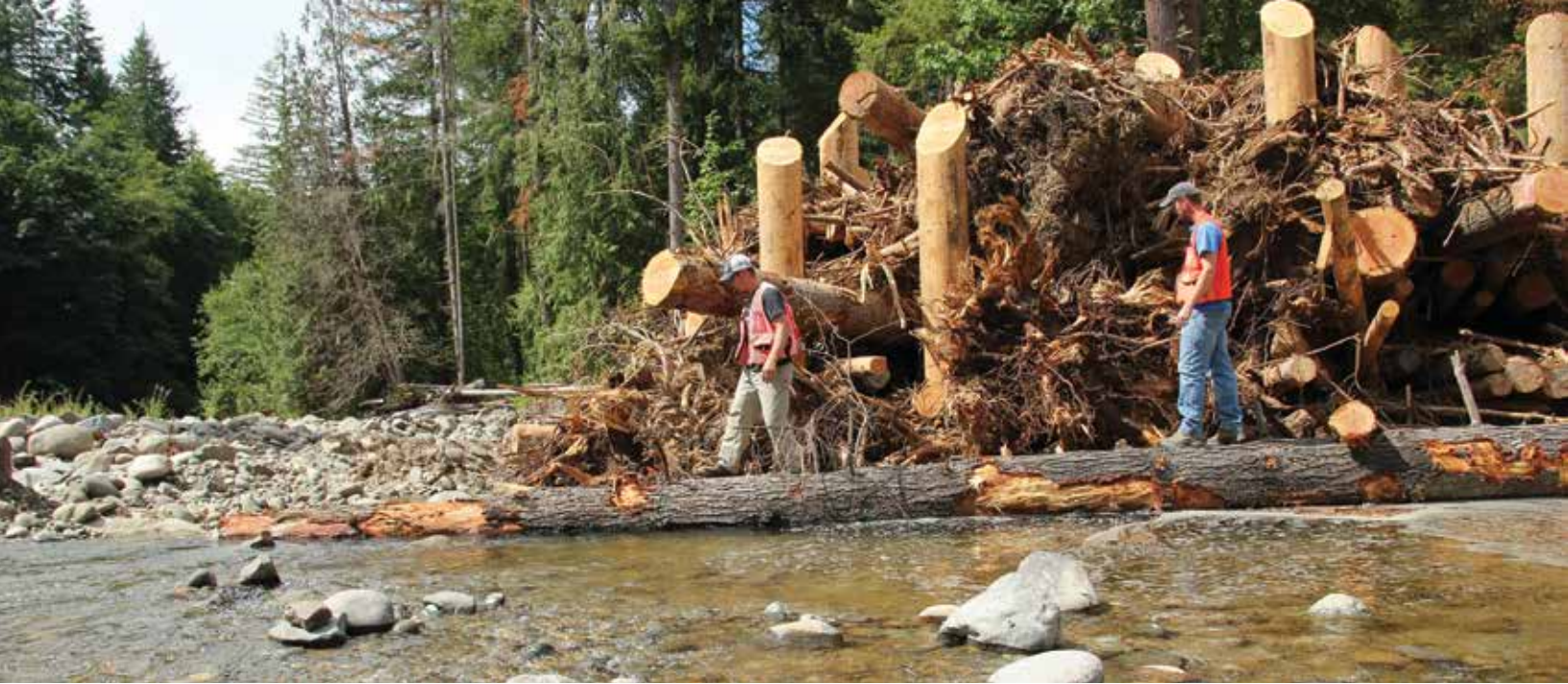
Nisqually Tribe natural resources technicians inspect an engineered logjam on the Mashel River. Emmett O'Connell
