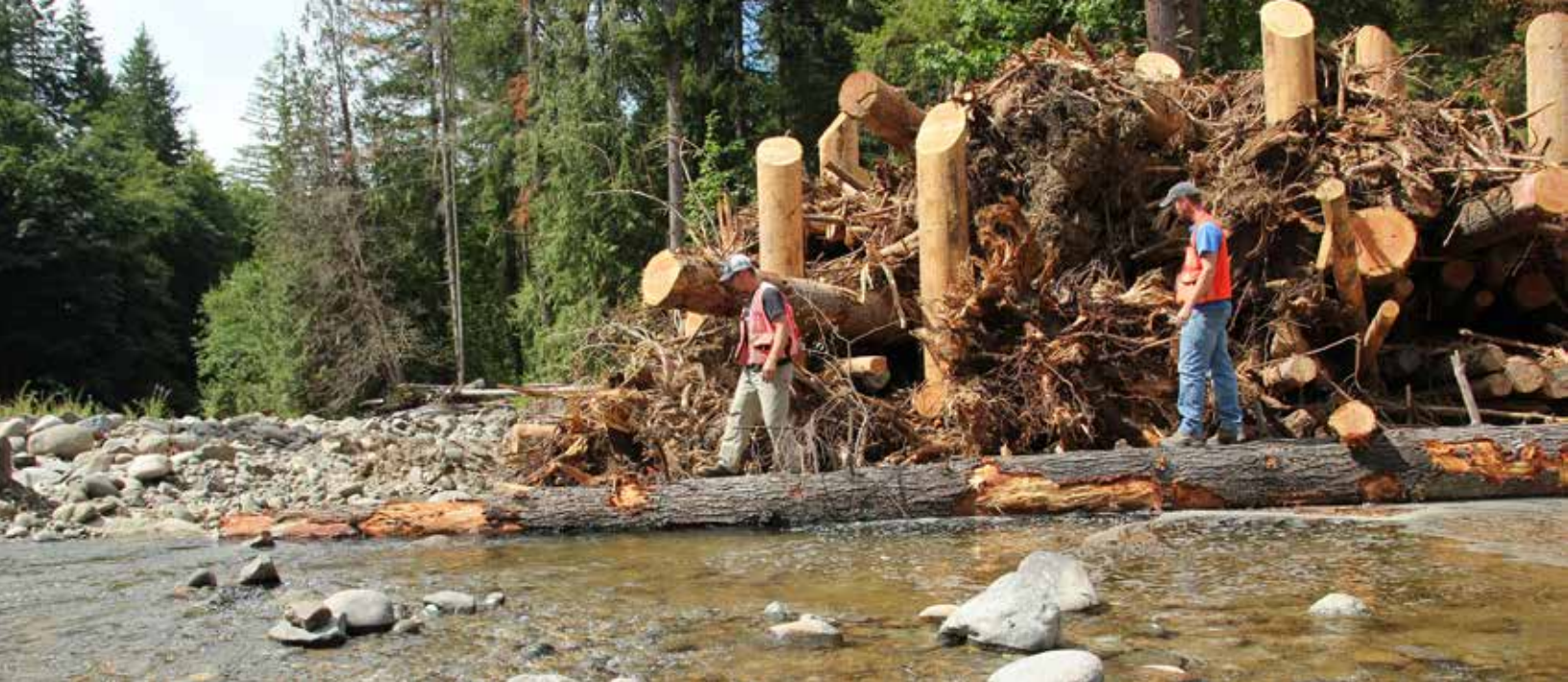
Nisqually Tribe natural resources technicians inspect an engineered logjam on the Mashel River. Emmett O'Connell
